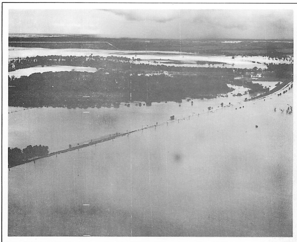
FIGURE I-24. Brazos River flood at Southern Pacific Railroad near Hempstead, Texas, May 1, 1957. Discharge about 140,000 cfs. Photograph by Corps of Engineers, U.S. Army.
