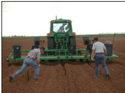
Figure 2. Installation of SDI laterals with GPS guided tractor, Joe Mustian, Doug Nesmith, and Cody Mull, TAES, 2005.
