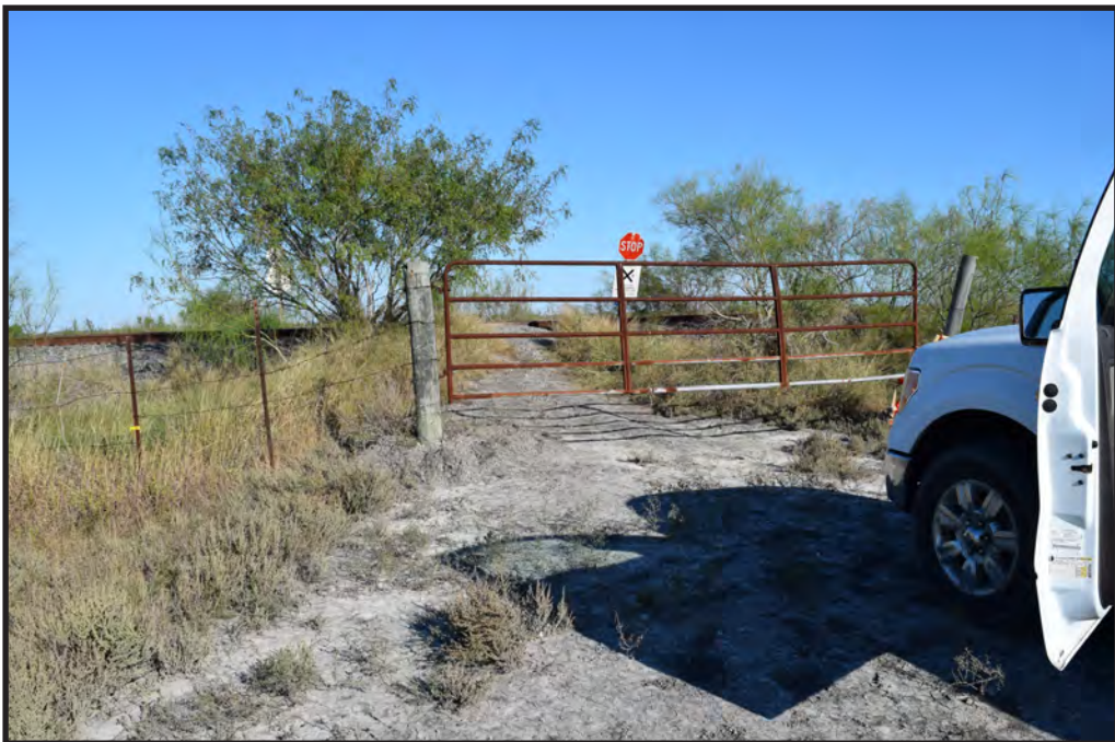
Photograph 2. Road #3 ends at the Union Pacific railroad track (looking east northeast).
