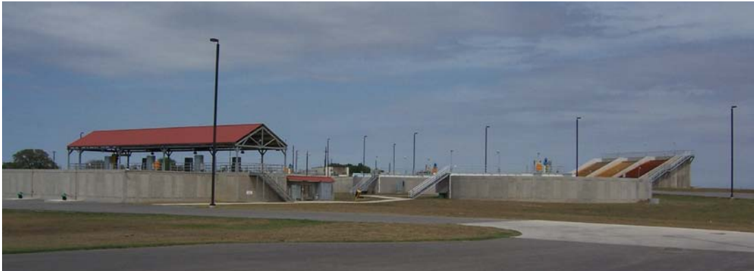
Figure 3-3: Water treatment plant (Morris, 2006)
