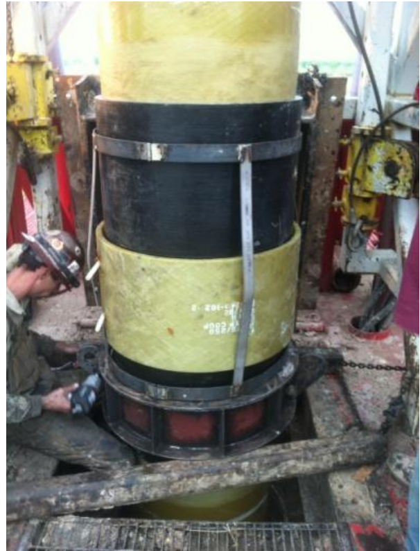
Centralizer installed around coupling Photo courtesy of RWH & Associates, Inc.
