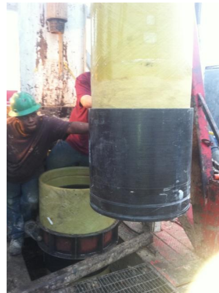
Casing installation Photo courtesy of RWH & Associates, Inc.
