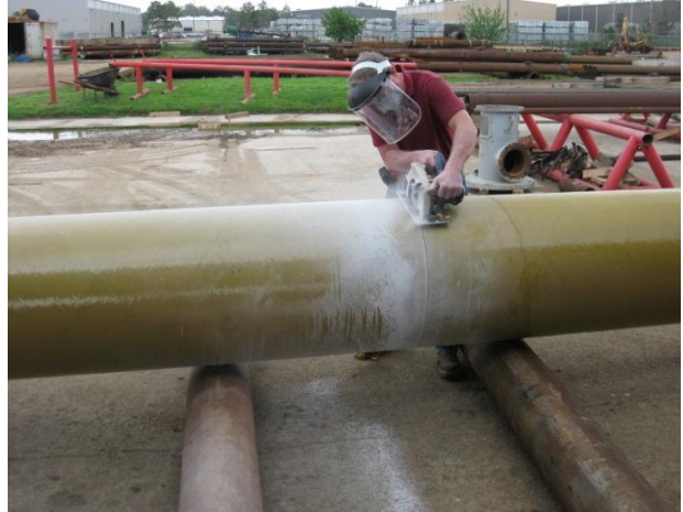
Cutting fiberglass casing Photo courtesy of Alsay, Inc.
