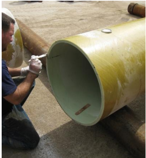
Application of epoxy resin Photo courtesy of Alsay, Inc.
