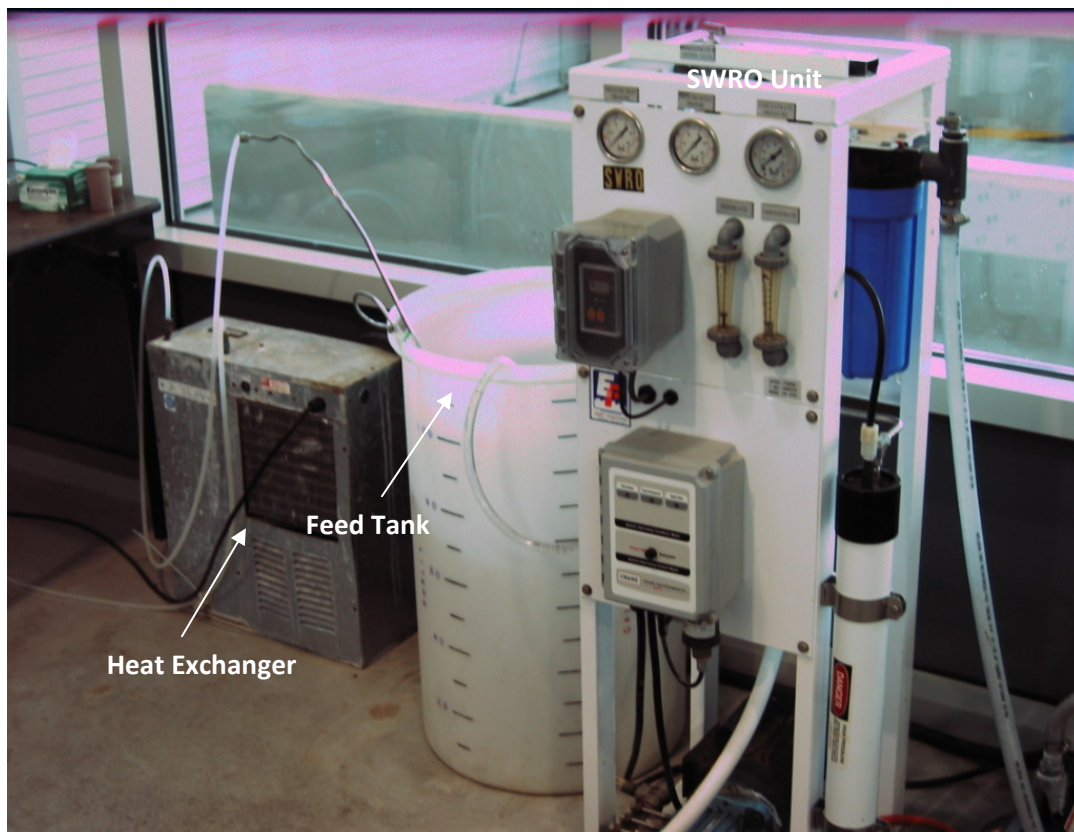
Figure 12. Picture of Small Seawater RO Unit Used for Conducting Initial Tests
