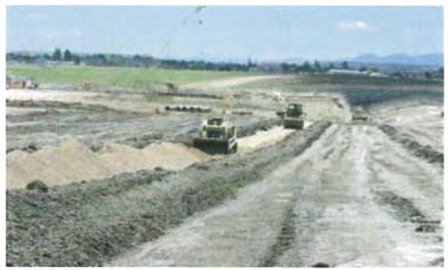
Vertical Chimney Drain Placement
