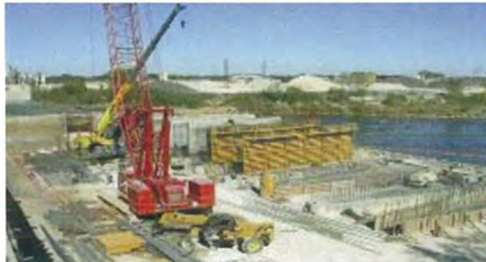
Labyrinth Weir Construction
