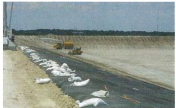
Soil Cement Anchor Trench & Liner/Curing
