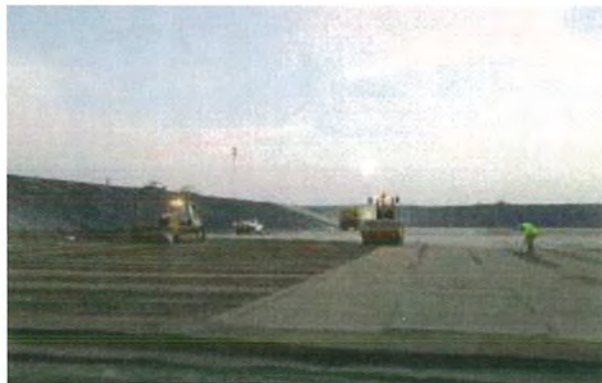
Soil Cement Placement
