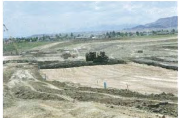
Zone II Clay Embankment over Blanket Drain
