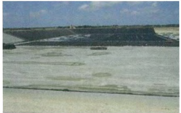
Reservoir Geocomposite, Liner, & Underdrain
