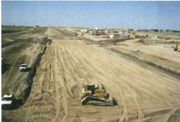
Downstream Sand Blanket (C-33)
