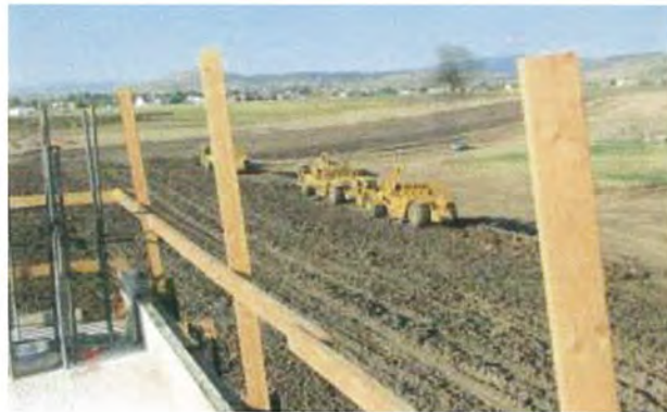
Zone I (clay core) at Embankment Interior
