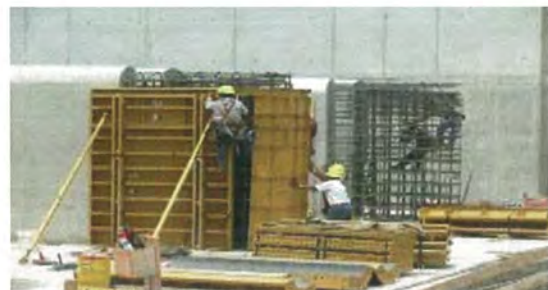
Apex Formwork & Reinforcement Installation
