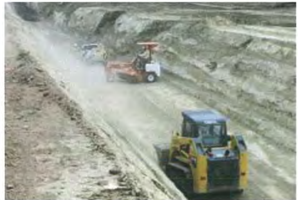
Core Trench Prep
