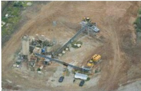
On-Site Soil Cement Plant
