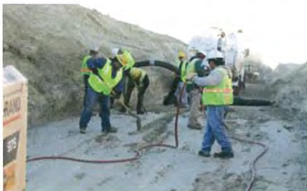
Core Trench Prep & Core Trench Slush Grout
