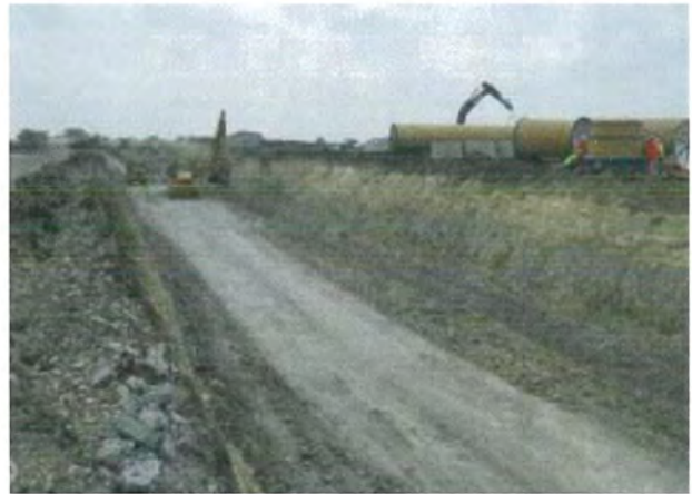
Excavation of Inlet/Outlet Piping
