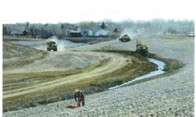
Care of Water and Spillway Bedding
