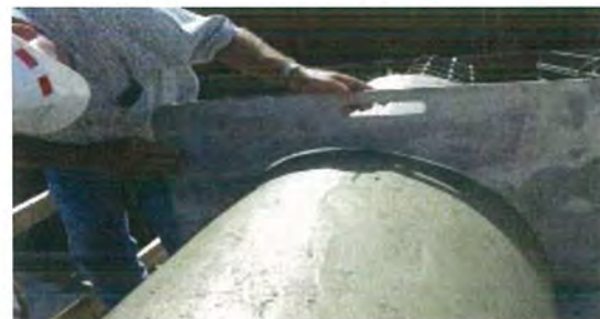
Crest Profile Check Finishing
