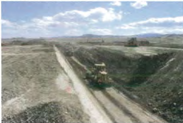
Core Trench Excavation/Foundation Prep
