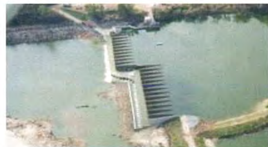
Completed Labyrinth Dam
