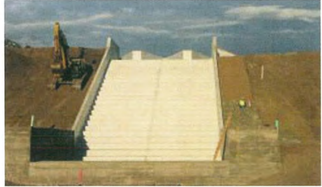
Completed RCC Emergency Spillway
