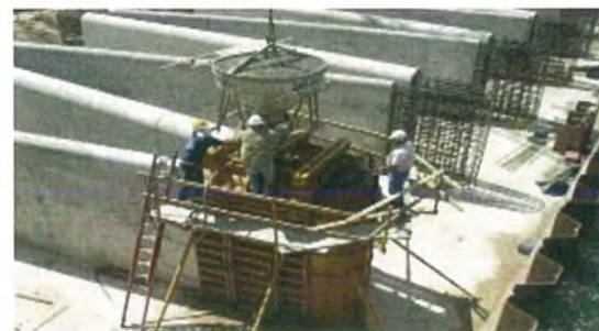
Apex Concrete Placement
